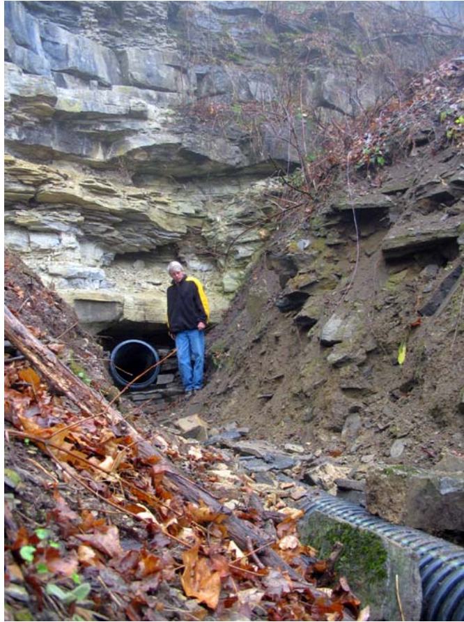
Culvert installation at Westfall Spring.
